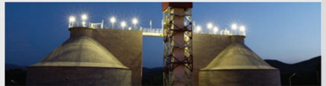
Sanandaj City Sewage Treatment Plant Sanandaj Waste Water Scheme
